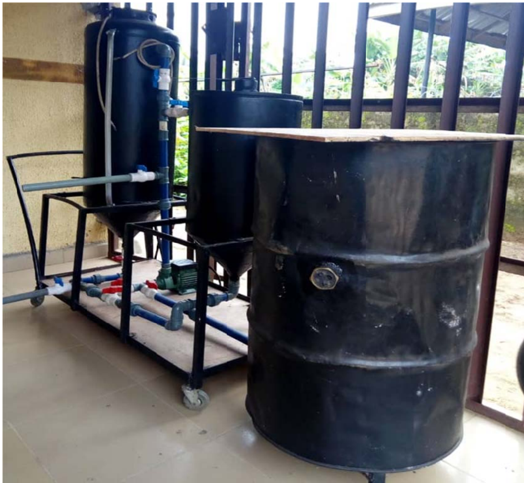
Figure 6: Completed Mini Biodiesel Production Plant
